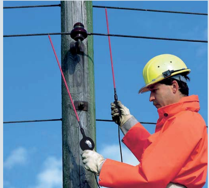
Two-pole SPN voltage detector used with extension prods for overhead lines
