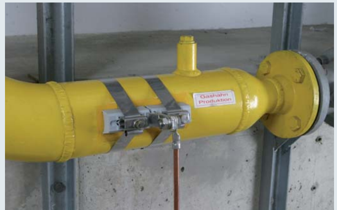
Pipe clamp for electrical contacting of pipes in hazardous areas for implementing of lightning equipotential bonding according to IEC/EN 62305-3 (EN 62305-3)
