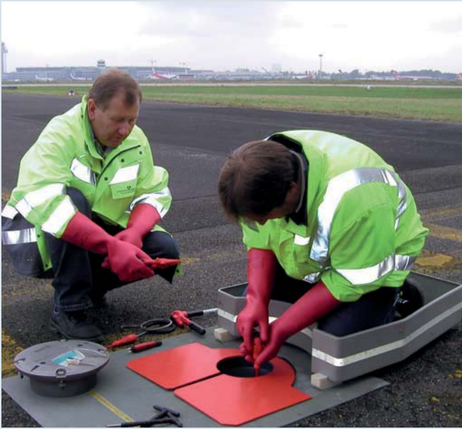
Replacement of a faulty illuminant (airport lighting system) at a runway
