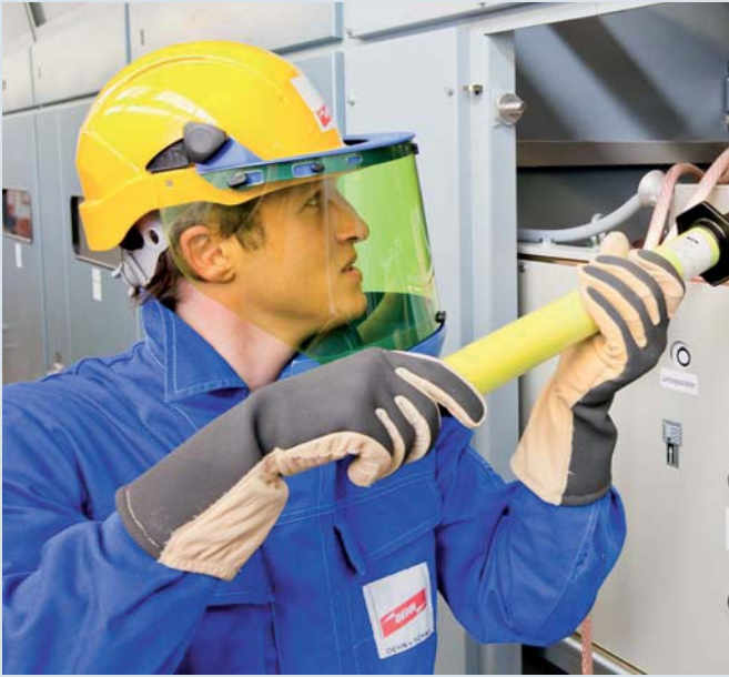
Attaching an earthing and short-circuiting device using the required personal protective equipment
