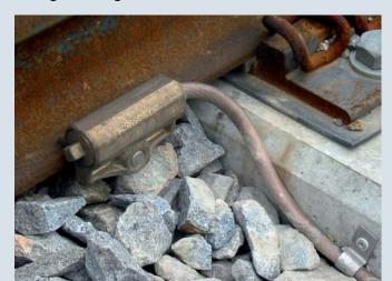
DIN EN 50122-1 describes the use of voltage limiting devices for d.c. and a.c. traction systems for so-called "open traction system earthing" of conductive components of overhead contact lines and current collectors. In order to prevent the occurrence of hazardous surges between the insulated tracks or track sections of electric railways and earthed parts of the installation, voltage limiting devices (SDS ...) are used.
