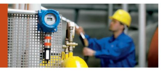
The Polytron FX is an economical, microprocessor-based gas detector for continuous monitoring of combustible gases and vapors in ambient air. Non-intrusive calibration and maintenance is performed using a magnetic wand to access the software through the enclosure window - no need to open the enclosure (and obtain special area permits) to perform routine calibrations.
