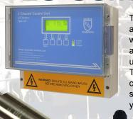
The 3000si and FGD3 is a wide range of sensors which are ATEX approved. These sensors are placed in the areas with the danger gases, in this case: NO, NO2, CH4, NH3 and H2S they then link to our control panel which allows users to view the status of each sensor simultaneously. The control panel also offers outputs such as relays which can be used to trigger extraction systems, beacons or system shutdown and 4-20mA which can be integrated into your BMS (Building Management System)
